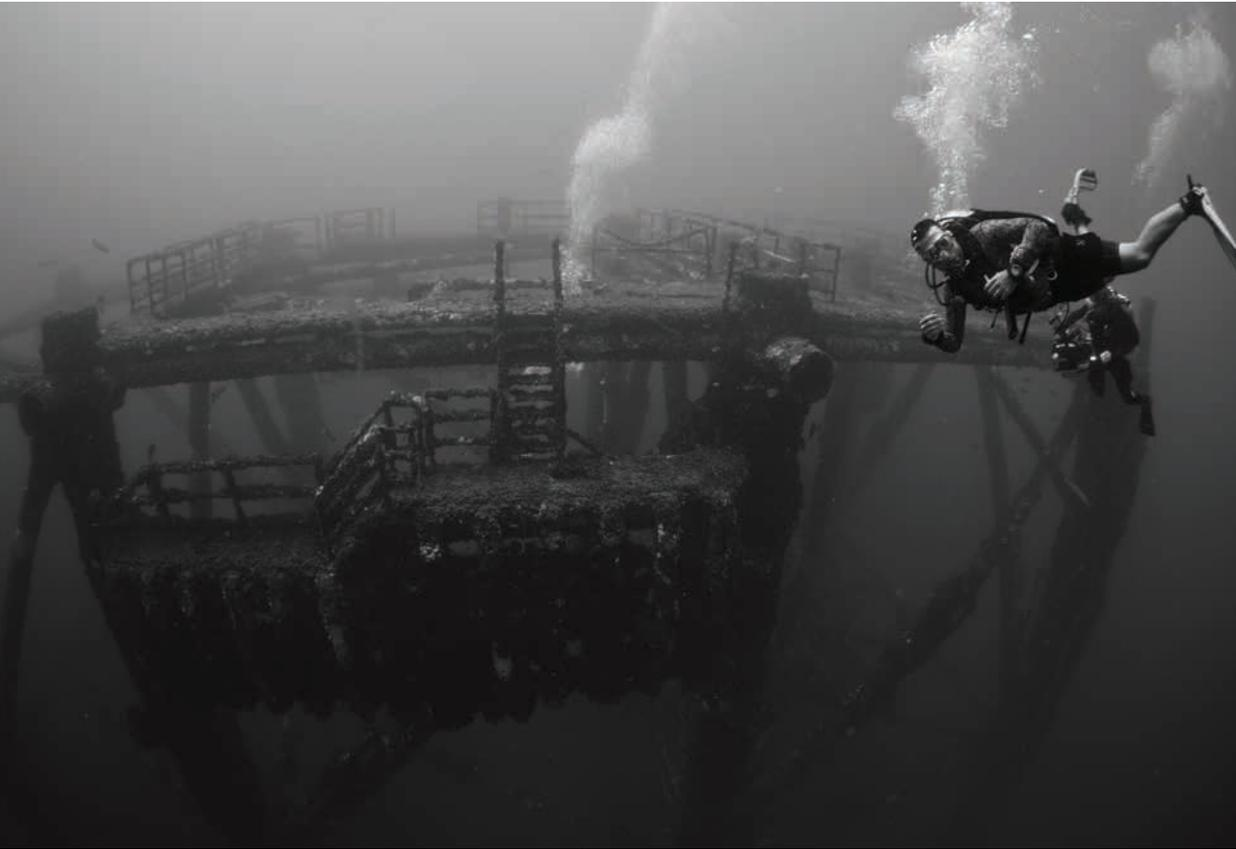
*This Rigs-to-Reefs deployment is at the High Island A-497 site, located 80 NM south east from Freeport, TX. The image shows the top of the structure which has been partially removed and placed next to the base. Image: Chris Ledford, Texas Parks and Wildlife Department Artificial Reef Program.*
