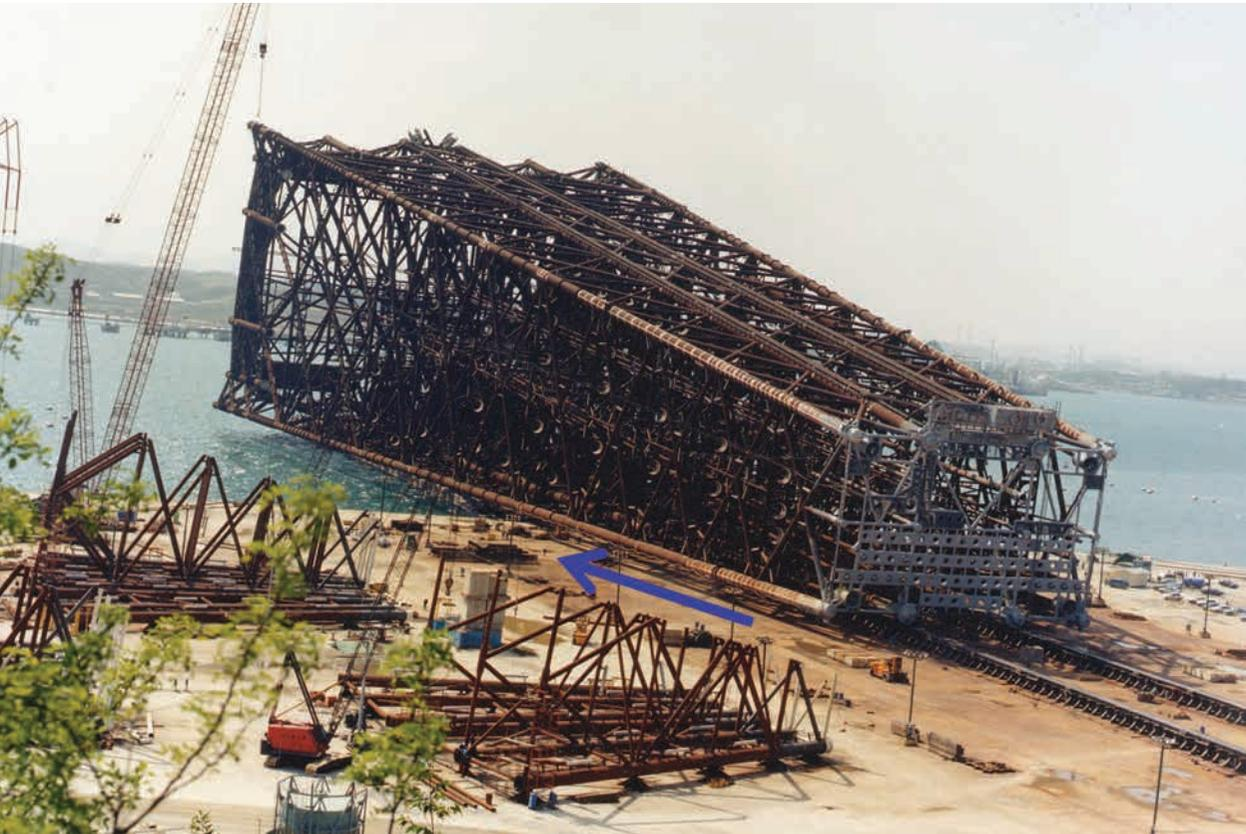
*A segment of the large ExxonMobil Harmony platform in 1998 onshore prior to its installation in California waters. For scale, the arrow points to a person.
